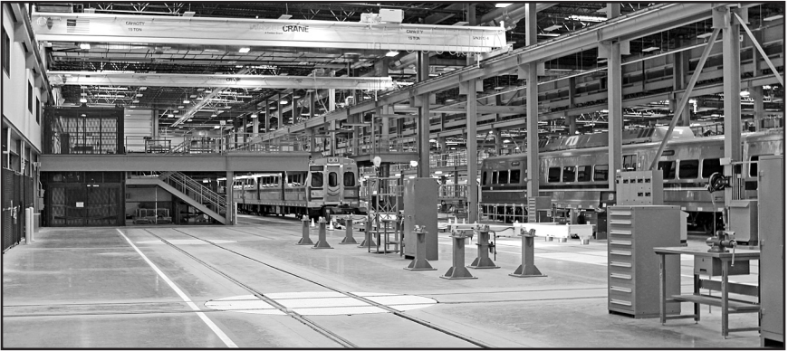
An opposite view from the photo on the previous page of the new RTD Commuter Rail Maintenance Facility on January 28, 2015. – Photo © 2015 Dave Schaaf.
